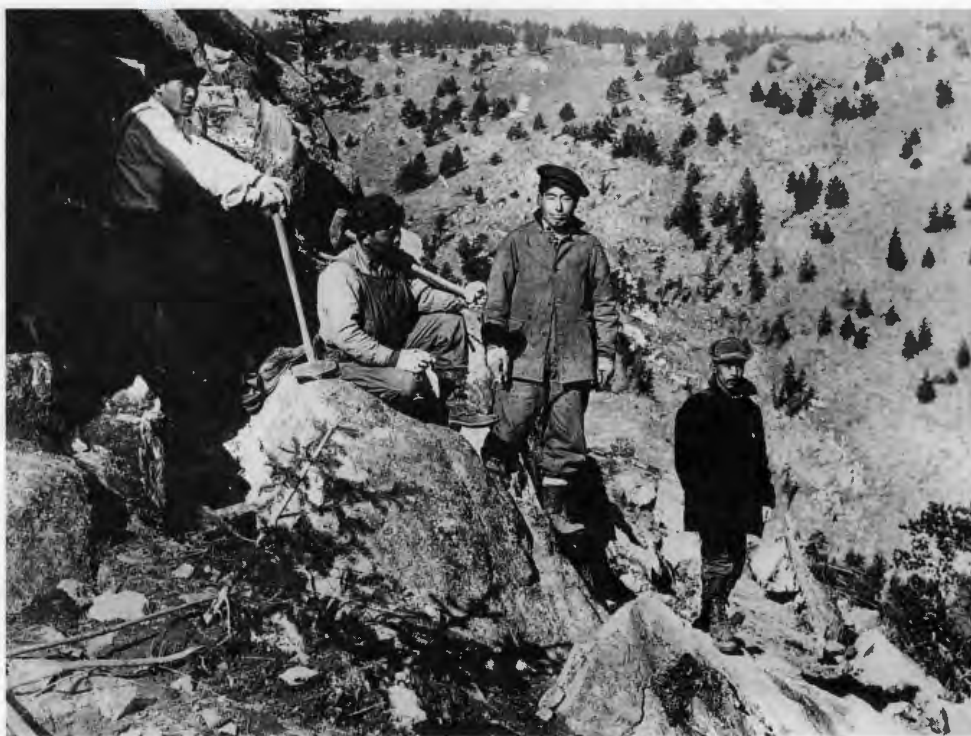
Japanese Workers Building a Road in California, c. 1910
